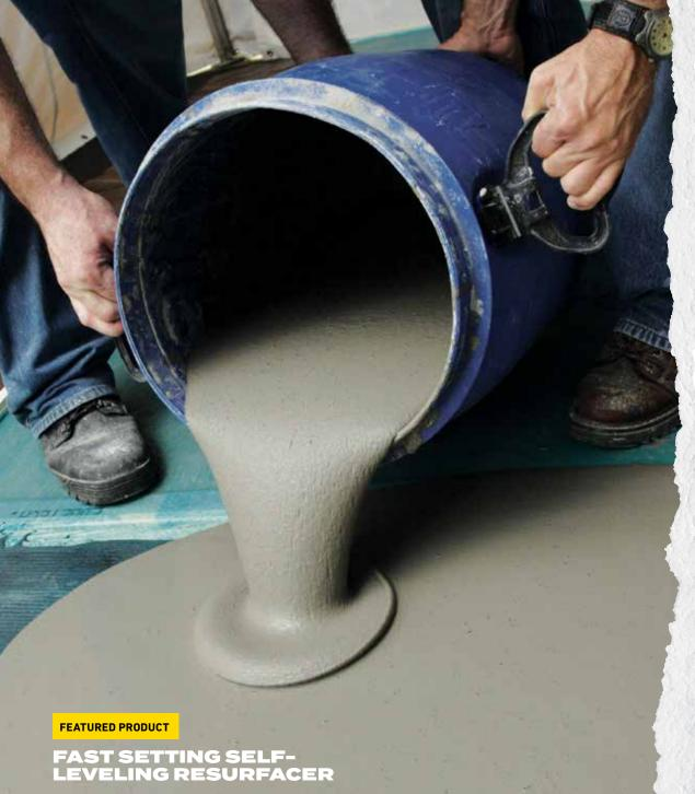
The only self-leveler rated for use as an underlayment or wear surface.
