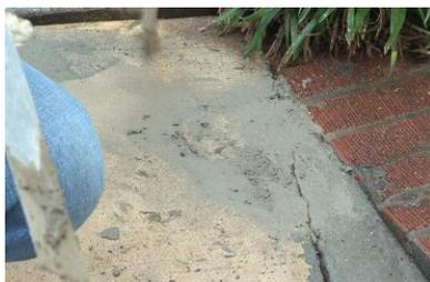
Use the finishing trowel to put a neat edge on the side of the repair and remove any excess material from joint areas.
