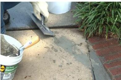
It may become necessary to use a finishing trowel and apply pressure to fill some of the voids.
