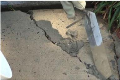
Using the margin trowel, place the material in the crack.
