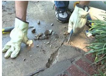
It may be necessary to widen the crack in some places. Once the area has been prepared, sweep away all loose concrete debris.
