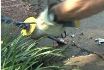
Clear out chipped, loose or unstable concrete from the repair area. This may require a hammer and chisel to break away the pieces.
