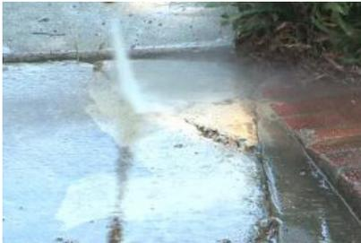
To ensure the area is adequately prepared for the repair, use a pressure washer or water hose to clean the area of dirt and surface build up. This step will contribute to obtaining a good bond between the existing concrete and the repair material.
